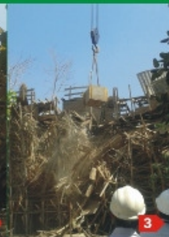
3 Breaking Crossflow Tower
