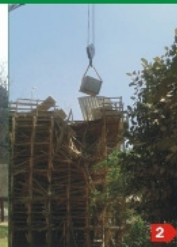
2 Breaking Crossflow Tower
